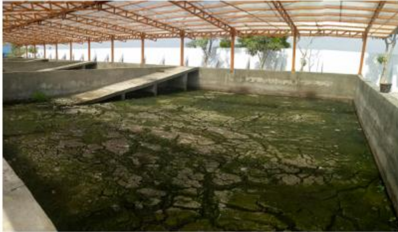
Gambar 1. Sludge separation chamber (SSC)
